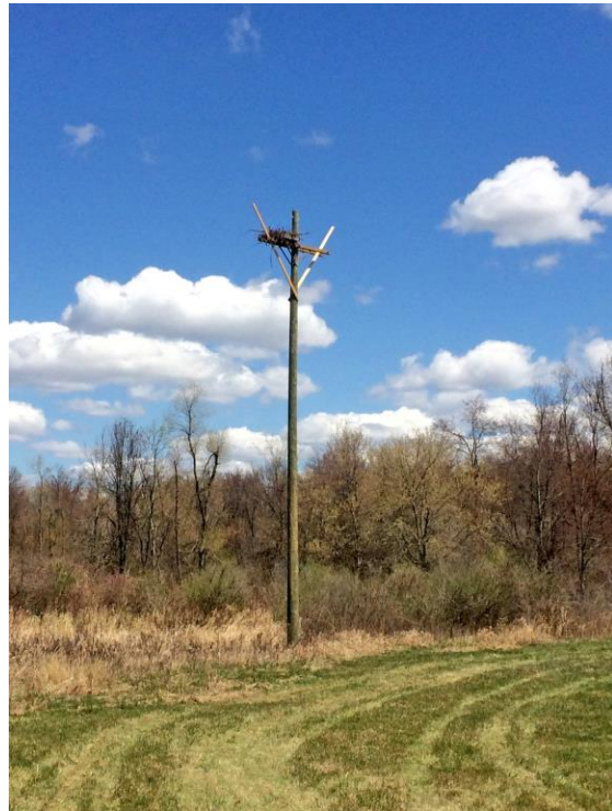
The new osprey tower in the North-80
